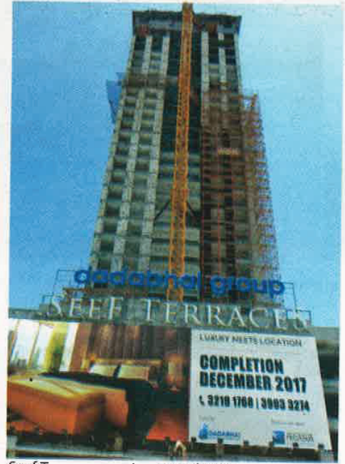
Seef Terraces nearing completion
